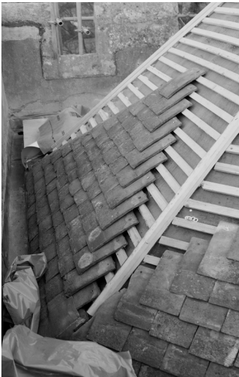
Tiles and battens
