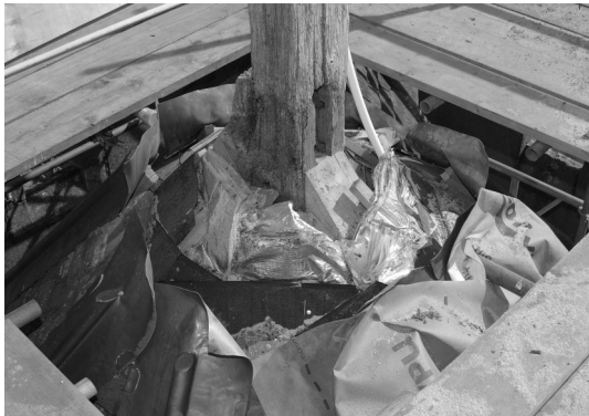
Layers on the roof, from the oak post to lead
