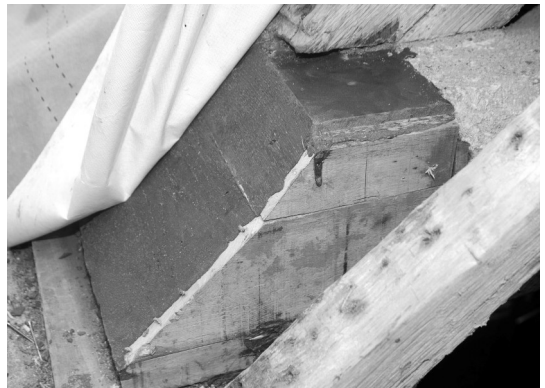
Painfully expensive Araldite on a tie beam
